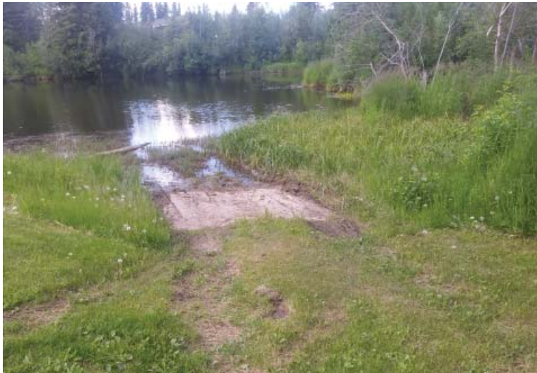
Noyes Slough Access - to be improved and made ADA accessible.
